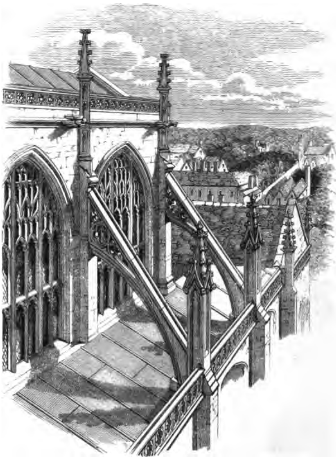
CLEERSTORY WINDOW AND ROOF OF SOUTH AISLE OF CHOIR FROM TOWER, LOOKING EAST.
